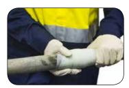
STEP 5: With wet gloves, squeeze the bandage with a rotating motion until resin stops foaming and is set. Allow a minimum of 30 minutes for Rapp-it Bandage to set rock-hard. For best results, ensure bandage application is at least 10mm thick.
