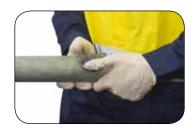
**STEP 2:** Knead Steel Putty and apply firmly into the damaged area. Putty has a 2-5 minute work time, and the bandage application must begin during this time.
