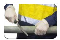
STEP 1: Shut down pipes or hoses. Apply gloves, then thoroughly clean and roughen the damaged pipe area. A clean, rough surface helps result in a successful repair.
