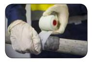
STEP 4: Quickly wrap the bandage around the damaged area, extending 50mm either side of the leak. Pull firmly throughout application.
